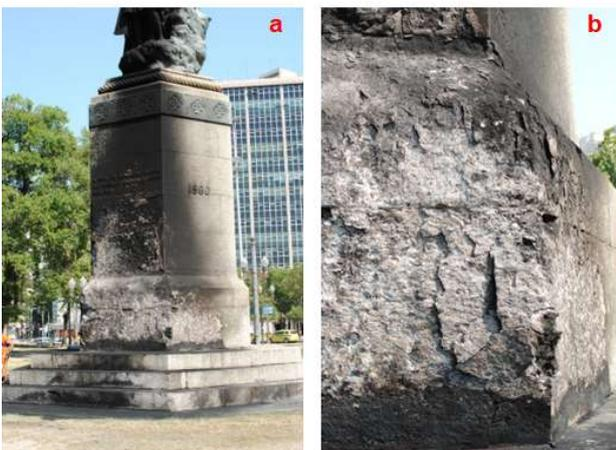
Figure 2: a) Monument aspect the day after fire and b) Detail of the damage. Photos by Pedro Dias.
